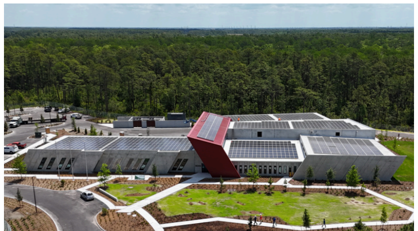
Solar panels on the newly built Fire Training Facility
