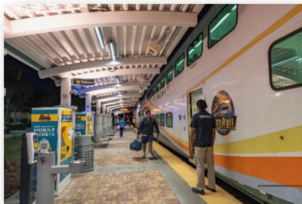
The lighting at the Sand Lake SunRail station was retrofitted with new LED lights, saving money on energy and maintenance
