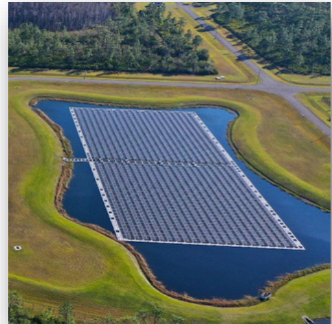
Orange County's floating solar array, located at the Southern Regional Water Supply Facility
