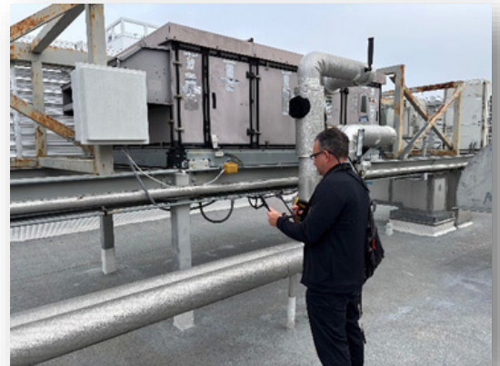
An Orange County building undergoing an energy audit
